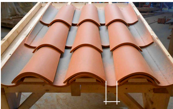
The gap between the tiles will be 20-50mm
