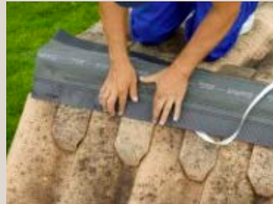
The ventilating ridge band (CAM01) is installed first on the ridge and stuck onto the upper part of the tiles and the wedges so that it is properly watertight.
