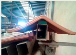
Q90 Ridge installation with Planum Tile (TI)
