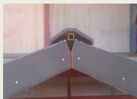
Q120 Ridge installation with Planum Tile (TI)
