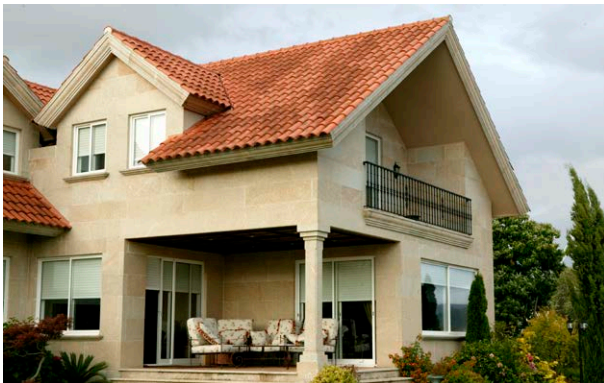
Humidity problems due to poor ventilation.
