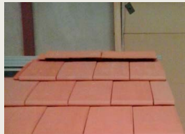
Q90 Ridge installation with Planum Tile (TI)
