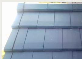
Q120 Ridge installation with Planum Tile (TI)
