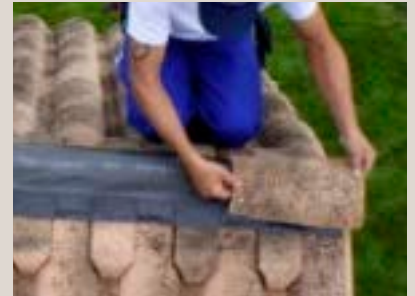
The ventilating ridge band (CAM01) is installed first on the ridge and stuck onto the upper part of the tiles and the wedges so that it is properly watertight.
