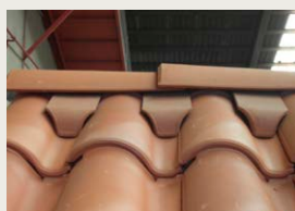
Q02 Ridge installation with Mixed tile (TG-TP)
