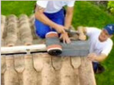
The ventilating ridge band (CAM01) is installed first on the ridge and stuck onto the upper part of the tiles and the wedges so that it is properly watertight.
