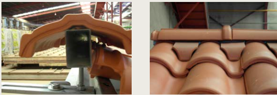
Q01 Ridge installation with Mixed tile TG-TP
